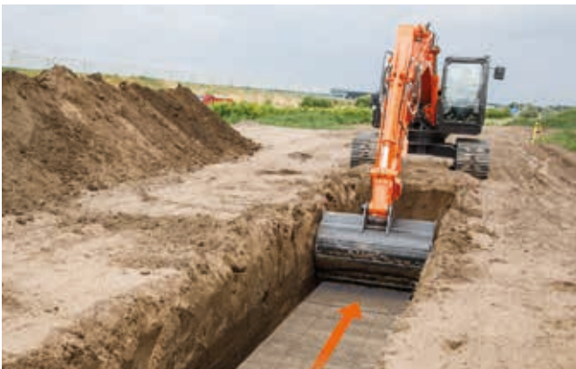
Trenches can be created efficiently using the overcut protection function.
