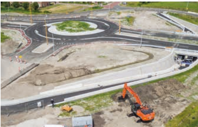
The 3D system identifies the actual position of the excavator.
