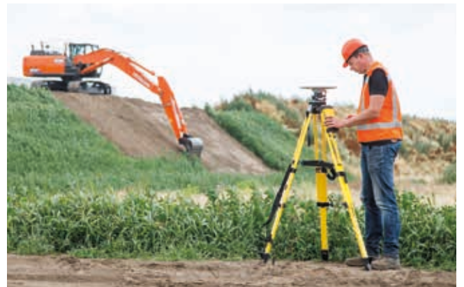
The machine receives 3D data via the internet or a USB device.
