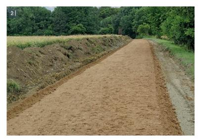
and mixing rotor. Soft soil is covered with lime spread by, for instance, a binder spreader prior to treatment. Subsequent homogeneous mixing by the milling and mixing rotor causes the lime to remove the excess humidity from the soil.
