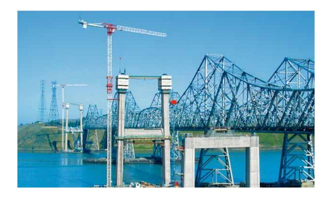
Tower cranes are most commonly used where the application not only requires height, but also reach. All four varieties of Terex® tower cranes give you the reach you need with the effi ciency that you want. Modular construction on most models helps reduce transportation costs.
