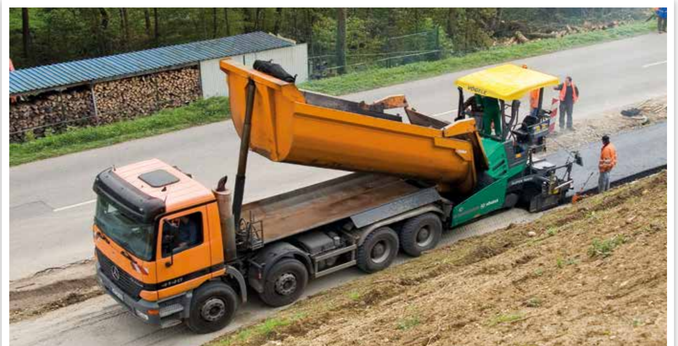
ASPHALT PAVING ON COMBINED FOOT AND CYCLE PATHS
