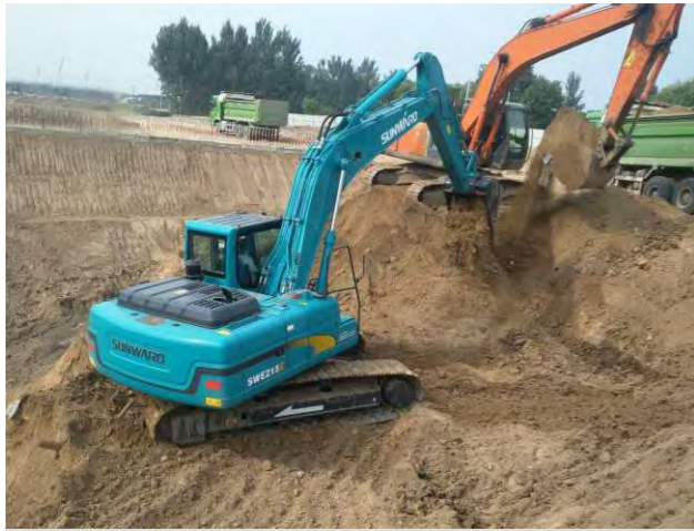
Construction by SWE215E in Beijing
