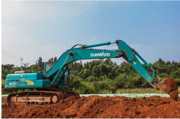
Construction by SWE235E-3 in Guangxi
