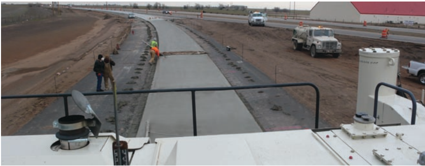
Excellent visibility of slab behind paver.
