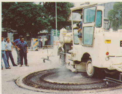
ROTO-MILL Profilers have a short turning radius for cutting around obstacles.
