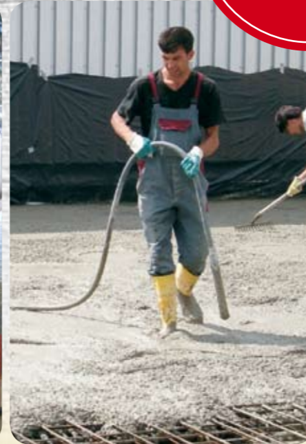
Step 6: The concrete should then be compacted. This gives it its top-class quality. The wide range of Wacker Neuson internal vibrators is ideal for this work.
