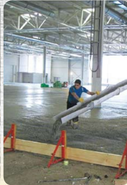
Step 5: The fresh concrete is delivered and poured.
