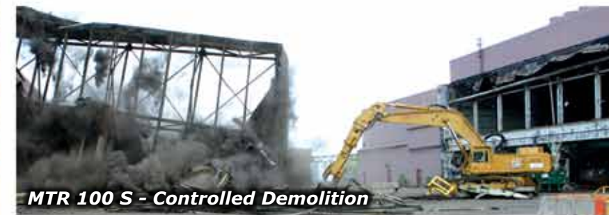
MTR 100 S - Controlled Demolition
