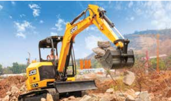
Construction site clearing
