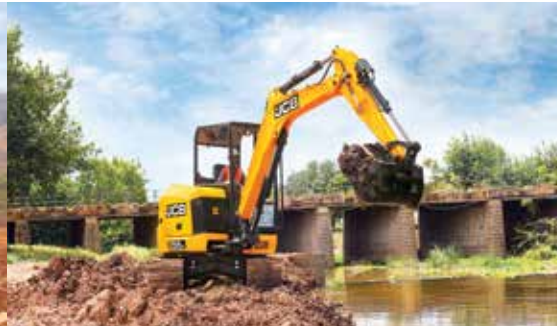
River bed re-building
