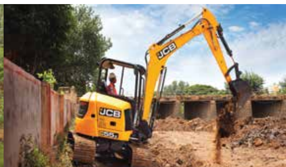
Digging close to wall
