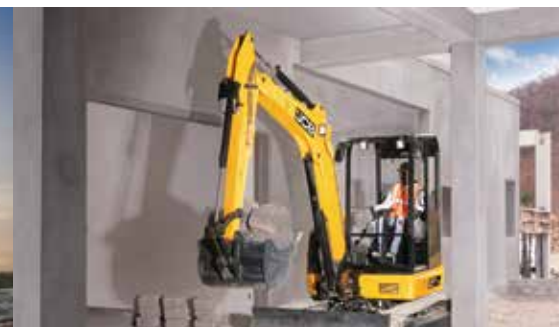
Building basement clearing
