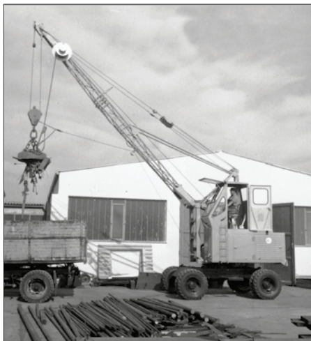
1962: rope-driven S833 with elevated operator cab
