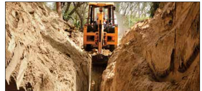
Trenching & pipe laying
